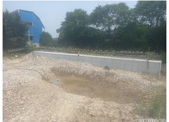
Sump formed next to the finished box culvert (R2)
