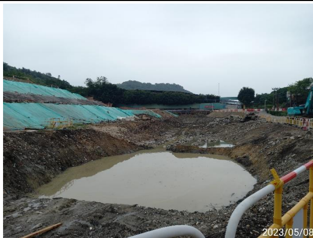
Temporary detention pond at the works area near the access road (R1)
