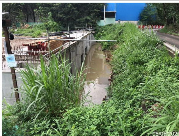
Water (mixed upstream river water and site runoff) detained temporarily behind the box culvert prior to treatment (R3)
